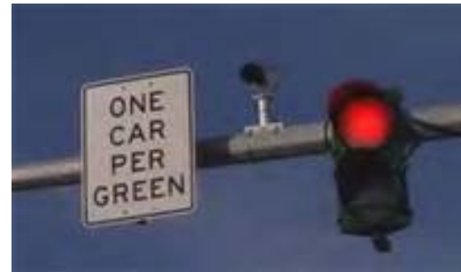
Figure 22. A ramp meter. (Source: Federal Highway Administration.)
