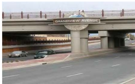
Figure 21. The new Grandview Bridge, “Gateway to Olde Arvada.”
